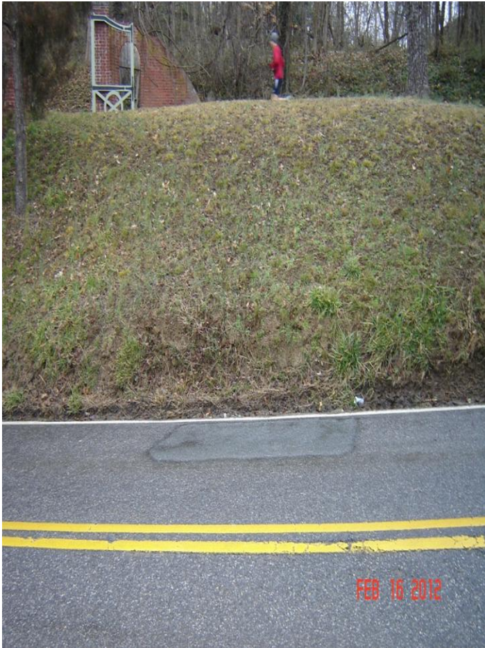
River Road Pothole Repair
