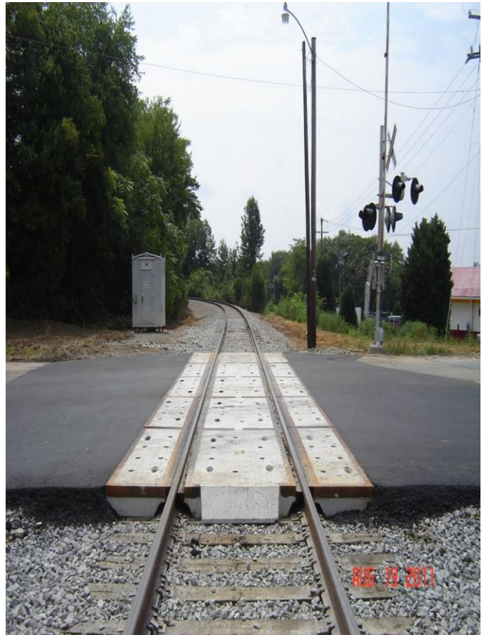
CSX Crossing (After)
