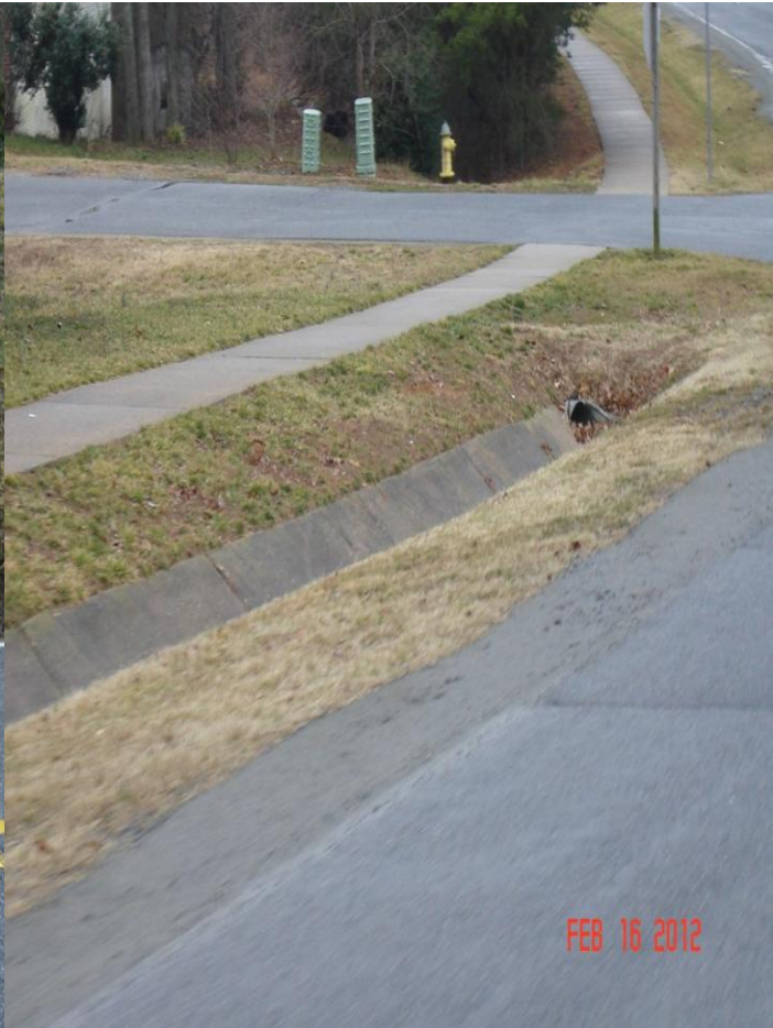
Cardinal Forest Shoulder Repair
