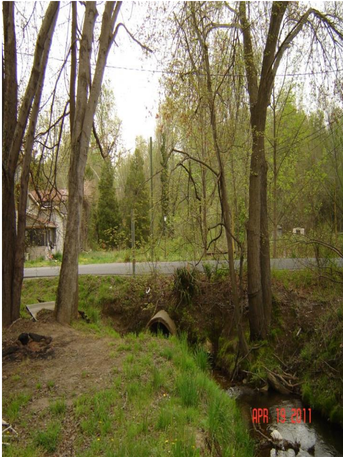
Decatur Road (Before)
