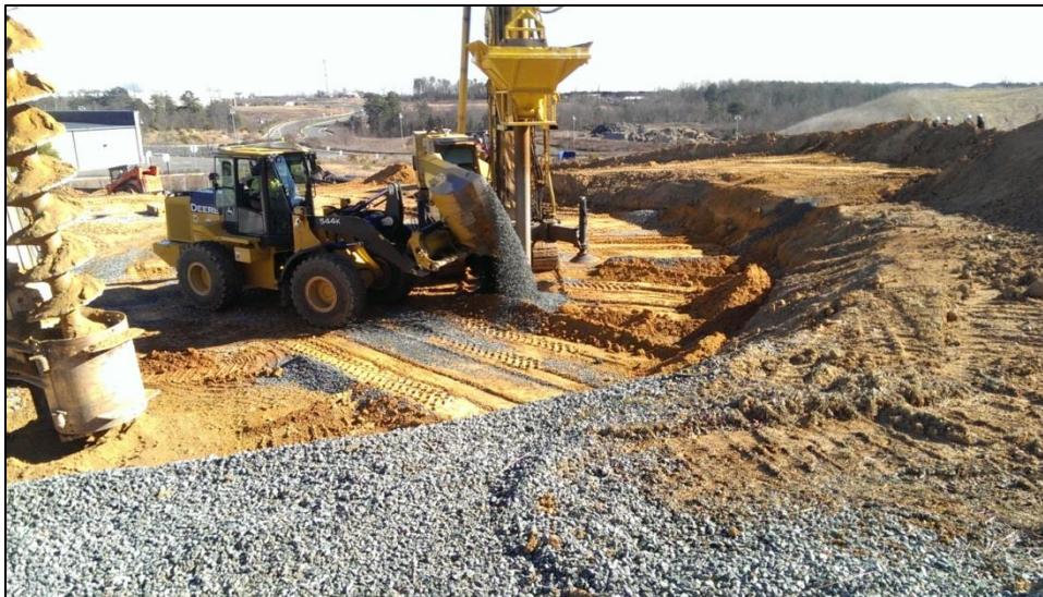
Installation of Vibra Piers to support the Water Tank
