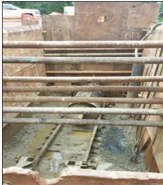
Bore operations to install sewer line under U.S. Route 1
