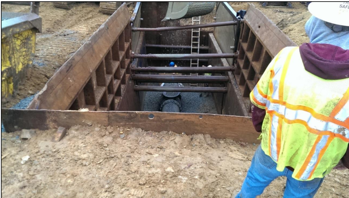
Installation of flushing tee near Rappahannock Landing
