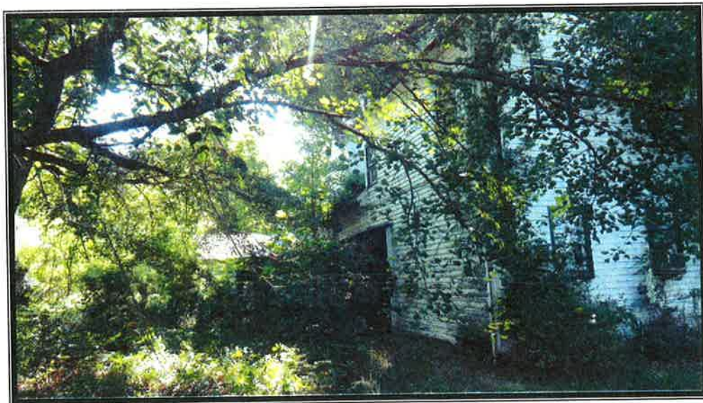
Plate 3. View of main house, side (west) elevation and rear (north) elevation addition, looking east.
