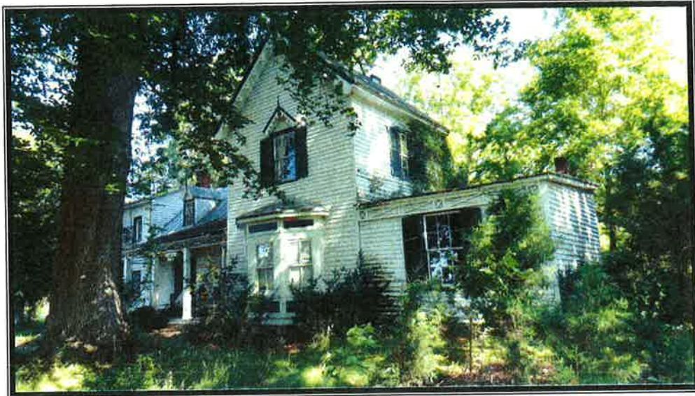
Plate 2. View of main house, façade and east elevation addition, looking northwest.
