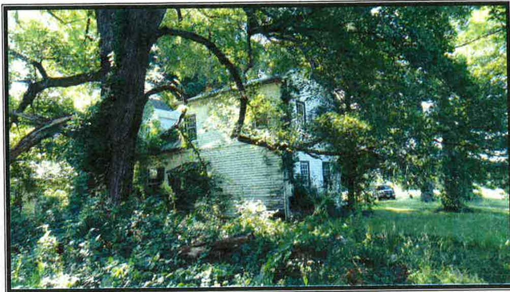
Plate 4. View of main house, side (west) elevation and rear (north) elevation, looking southeast.
