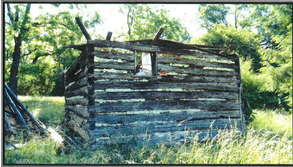
Plate 14. View of school, side (north) and rear (west) elevation, looking east.
