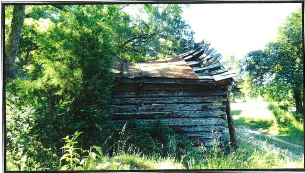
Plate 18. View of corncrib, rear (north) elevation, looking south.
