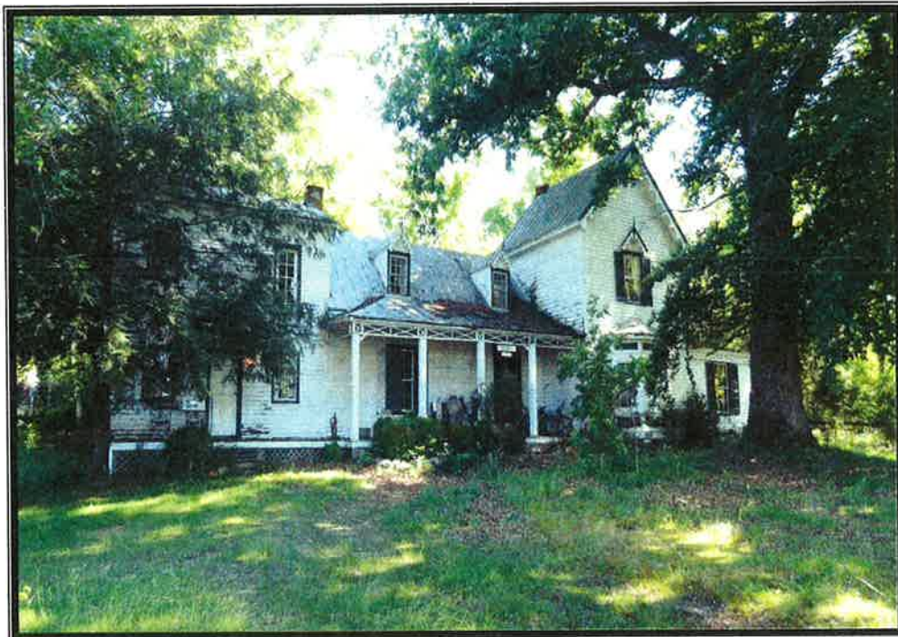
Plate 1. View of main house, façade, looking north.
