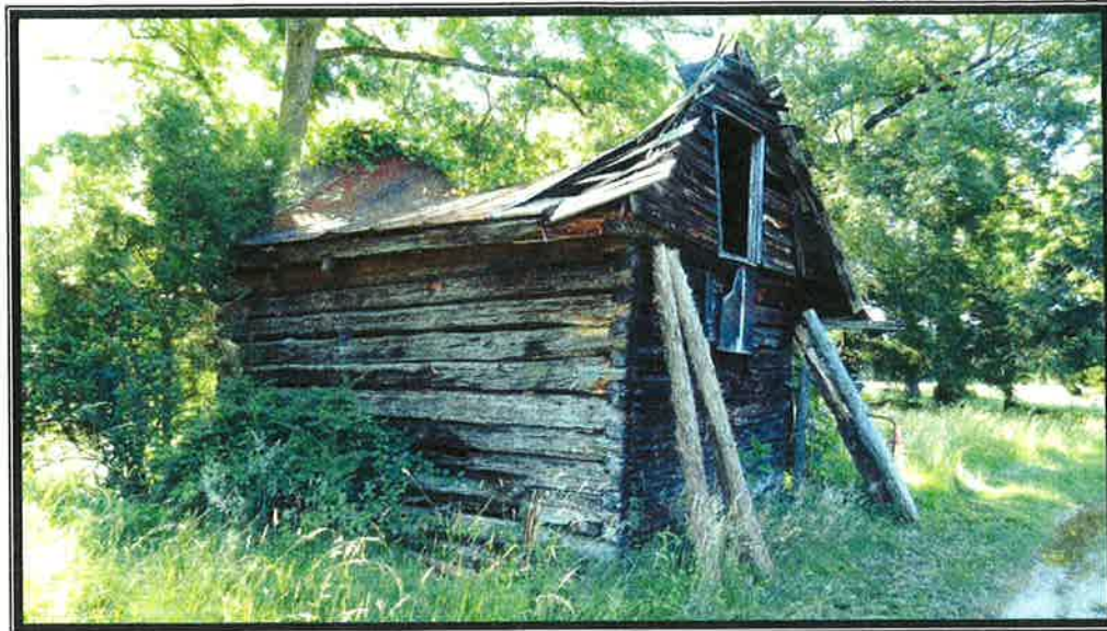
Plate 20. View of corncrib, rear (north) elevation and side (west) elevation, looking southeast.
