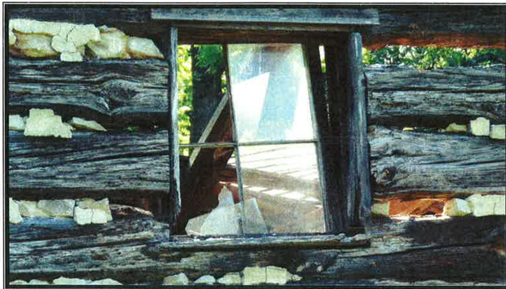
Plate 15. Detail view of school window.
