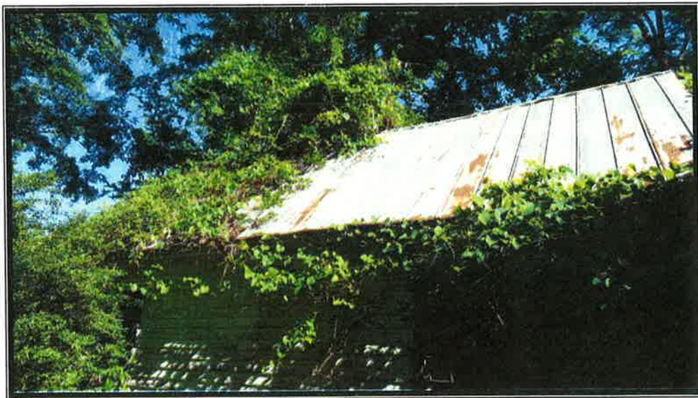
Plate 9. View of kitchen, side (south) elevation, looking northwest.
