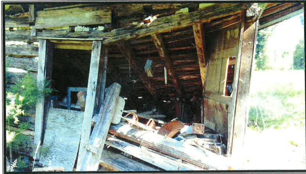
Plate 16. View of school, side (south) elevation and interior, looking north.
