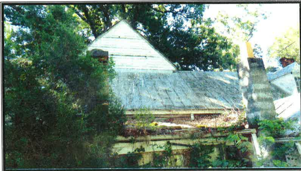
Plate 7. View of main house, roofline of rear (north) elevation addition, looking south.
