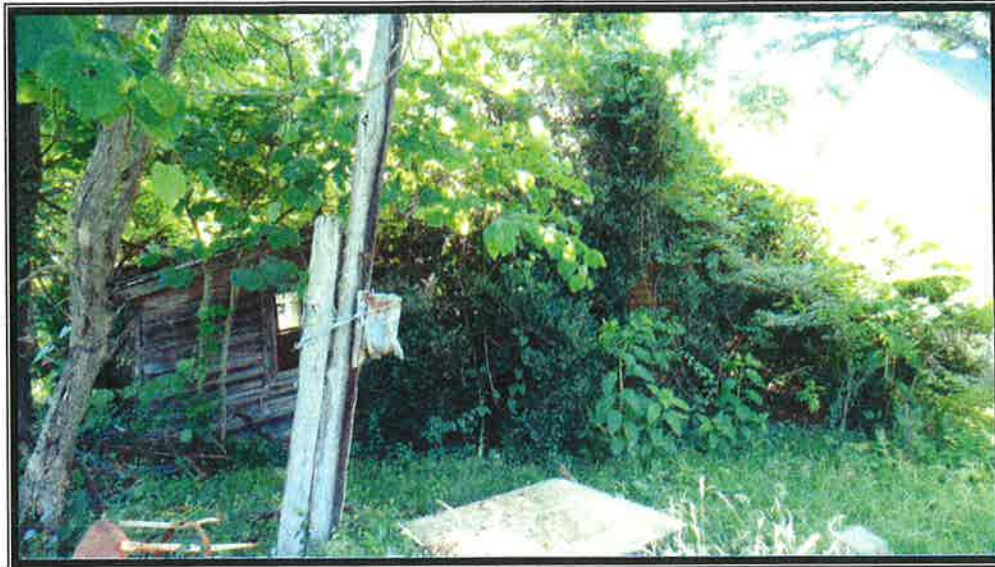
Plate 10. View of kitchen, side (north) elevation addition, looking east.
