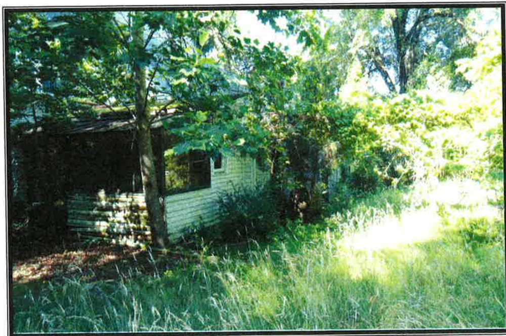
Plate 5. View of main house, rear (north) elevation additions, looking southeast.
