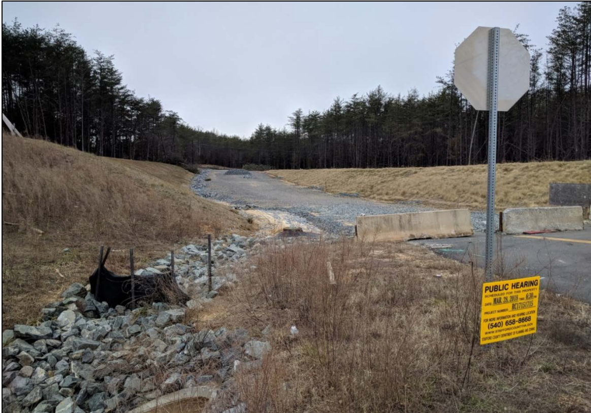
View from Centreport Parkway showing the existing access road
