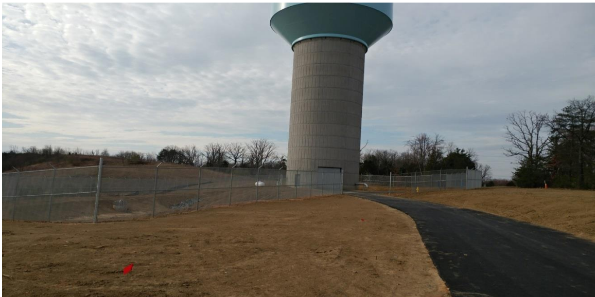
New Tank in Operation – Site work complete awaiting stabilization
