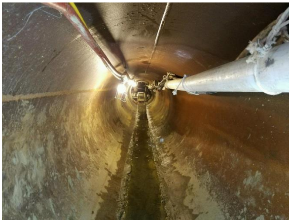
Looking upstream at rear of Tunnel Boring Machine
