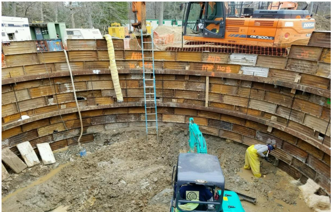
Microtunnelling/Boring Shaft Construction
