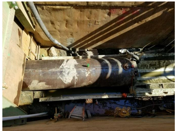
Looking into bore pit as the casing pipe is installed
